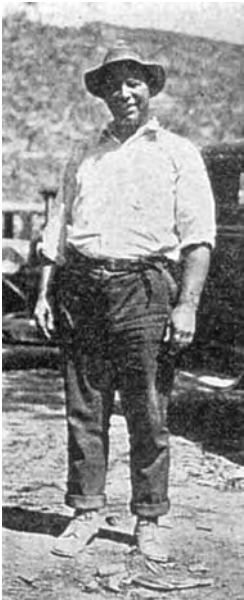
Robert G. LeTourneau at the Santiago Creek Dam, Orange County, California in 1931. He was general contractor on this job and his telescopic scrapers meant the difference between finishing the job on time or not at all. Western Construction News.
